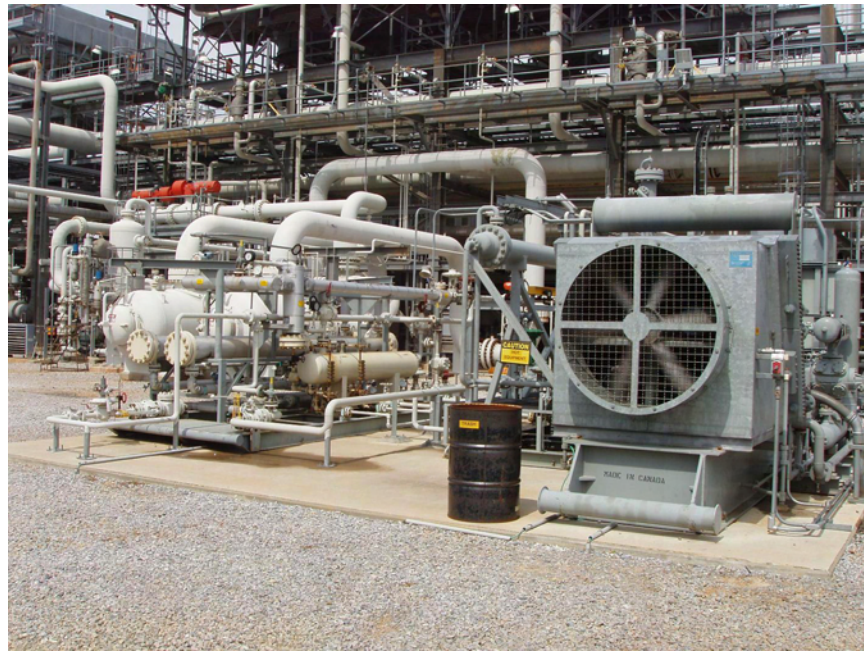
Figure 5. Membrane pilot skid and compressor skid at BP Amoco Pascagoula, MS, natural gas processing plant site.
