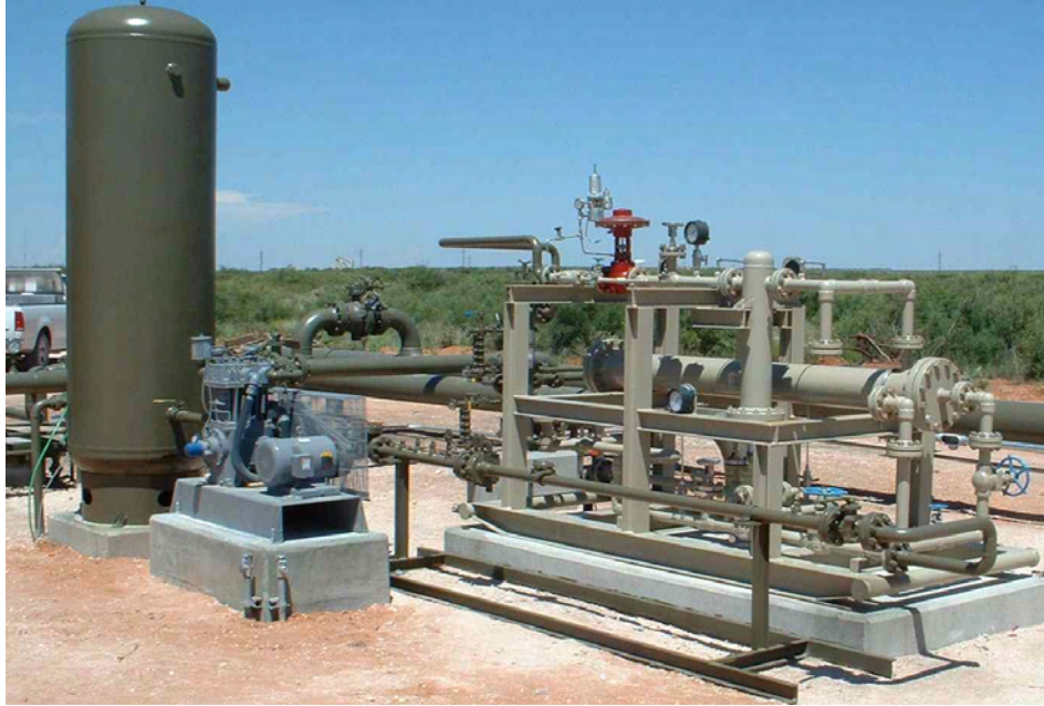
Figure 12. Membrane-based FGCU installed at one of Sid Richardson Company’s compressor stations in New Mexico.
