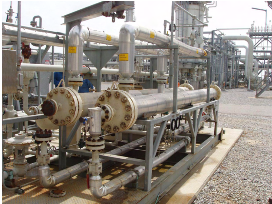
Figure 7. Rear view of membrane pilot unit in Pascagoula, MS.
