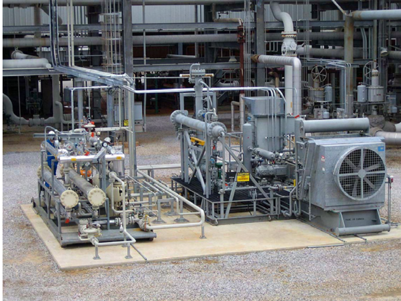
Figure 1. MTR's field demonstration membrane-based gas treating unit at BP Amoco's gas processing plant in Pascagoula, MS. The unit operated virtually continuously from December 2005-September 2006.
