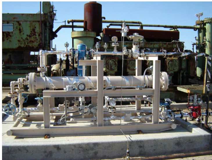
Figure 14. FGCU for an oil exploration firm, used at a California site to reduce total emissions and improve engine performance (Customer F).
