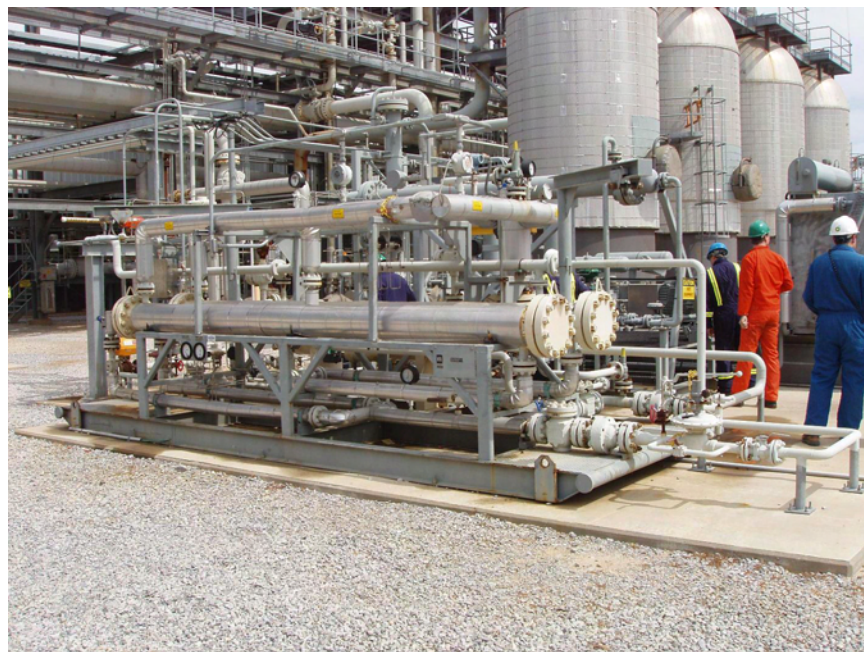
Figure 6. Membrane pilot unit – side view prior to final installation.
