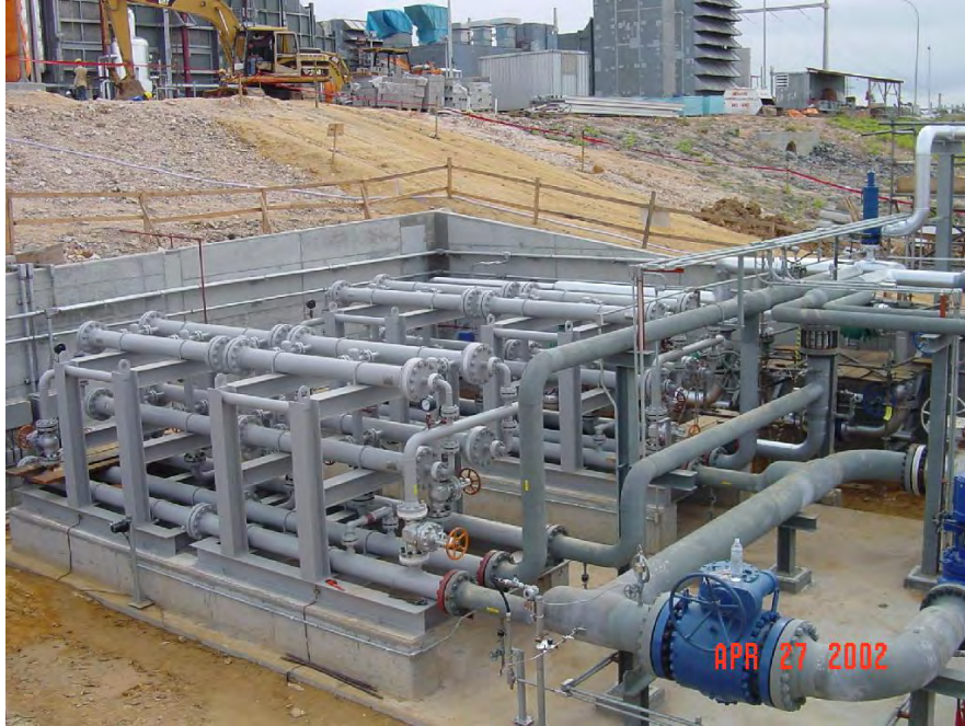
Figure 11. FGCU skids built to remove heavy hydrocarbons from onsite gas used as fuel for two 250 MW Siemens power plant turbines in Curitiba, Brazil. The unit was built on two identical compact skids so that the equipment could be shipped easily by air.
